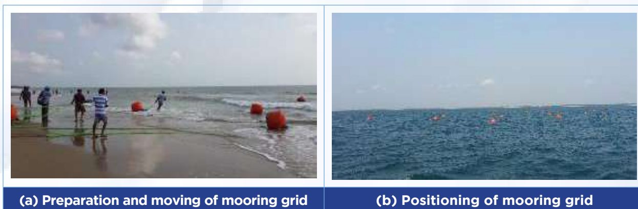
Figure 39. Mobilization and positioning of mooring grid
