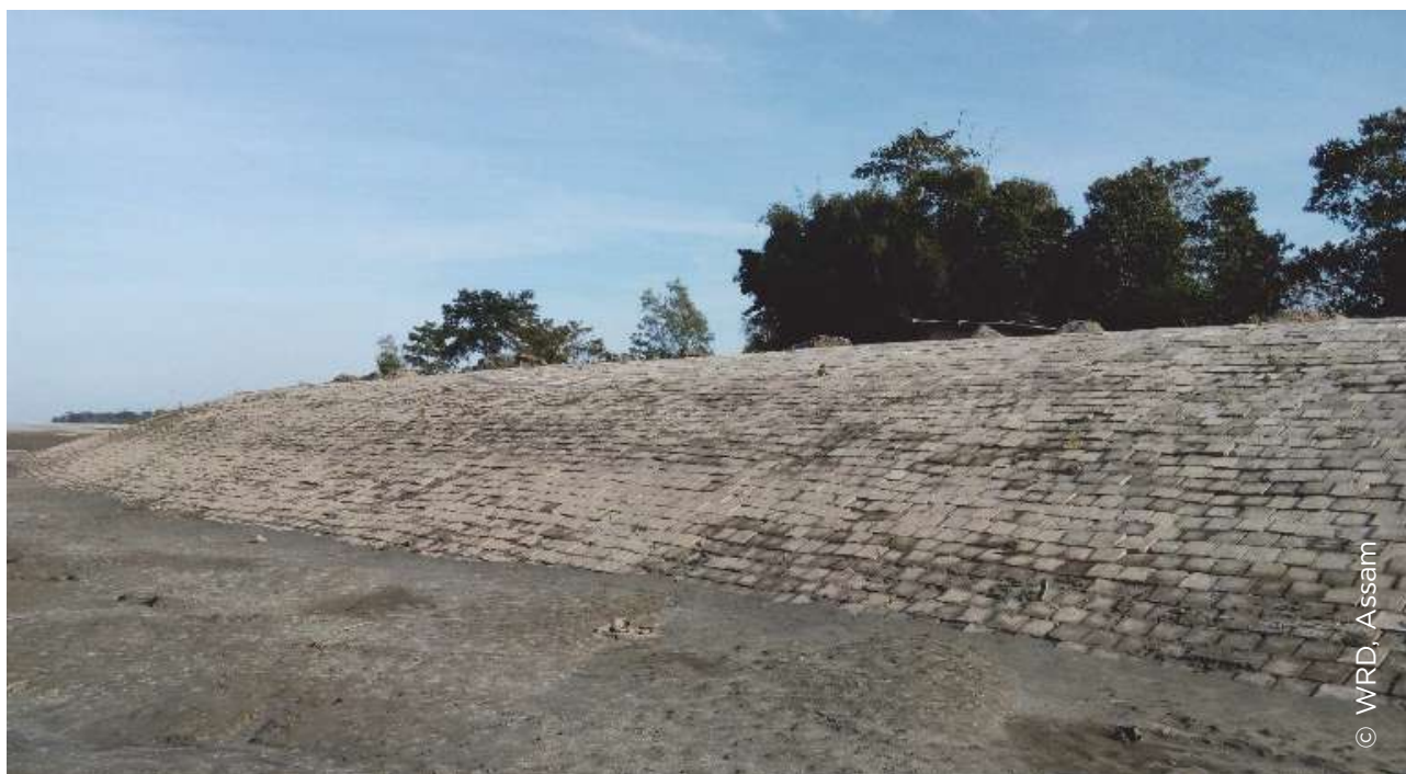
Use of CC block revetment on dyke
