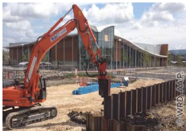
Construction of Sub Surface dam through Z sheet piling
