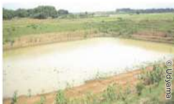
Community Tank Renovation
