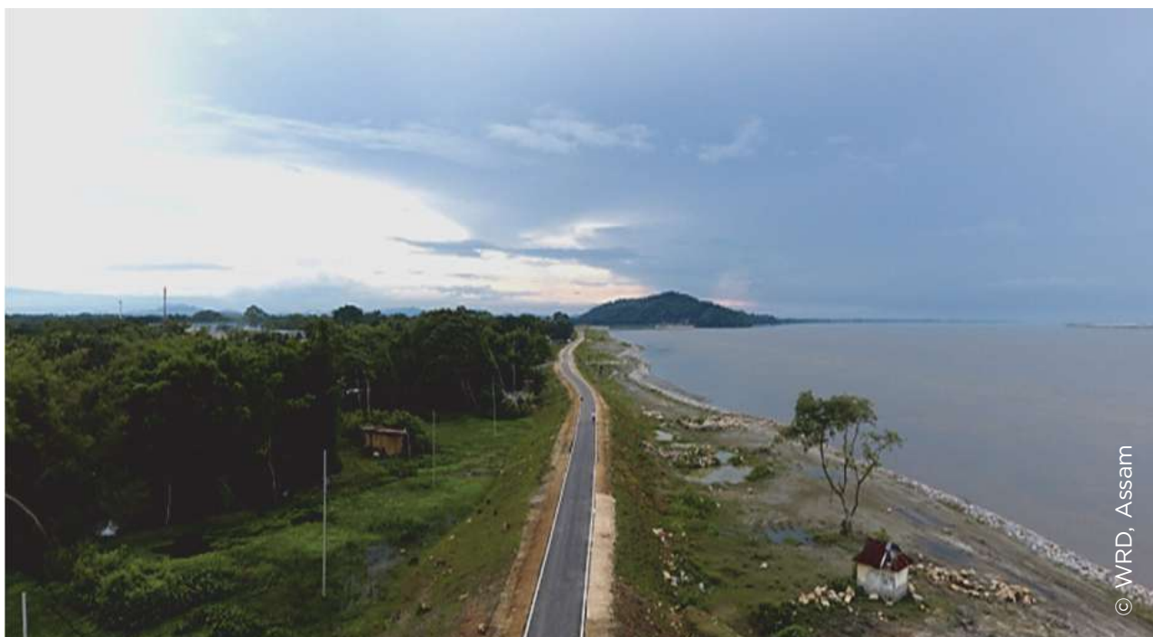
Embankment cum Black Topped Road
